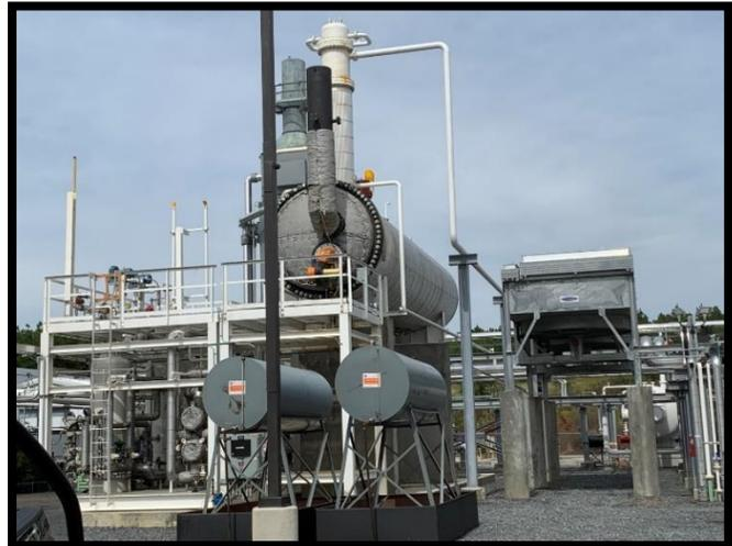
Consider the following example: A local operator finds that a glycol heater will not restart after a system trip. Fortunately, the local heater control panel was supplied with an intuitively-obvious graphical indication and/or display verbiage that the low fuel gas pressure switch is in alarm. A simplified graphic, such as the one pictured below, easily identifies the low fuel gas pressure switch as “below limit.”
